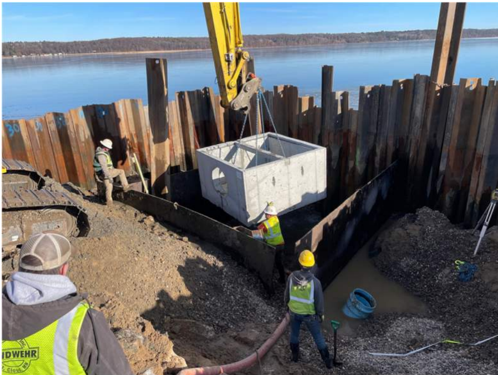
Photo #5: Setting inlet structure - Nov 29, 2023, 11:23 AM
