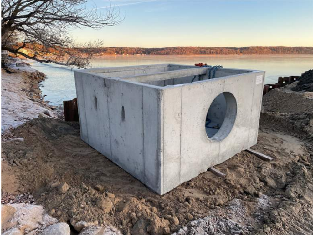
Photo #4: Inlet structure delivered - Nov 29, 2023, 7:57 AM
